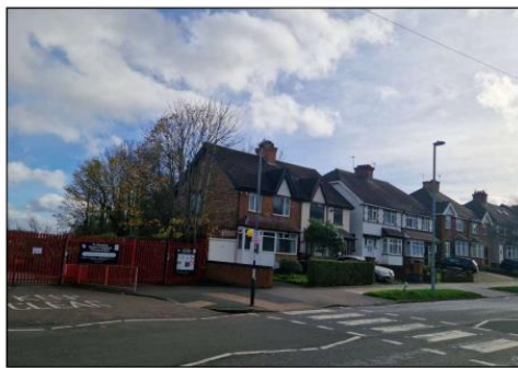
Existing Site Photograph
